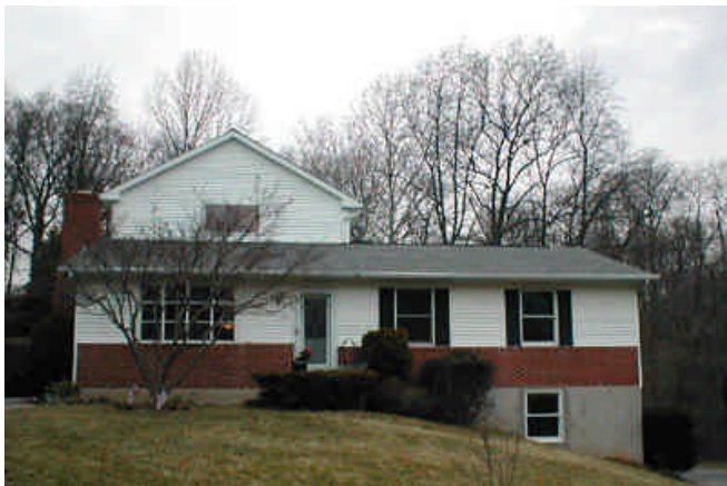
Front façade, before
