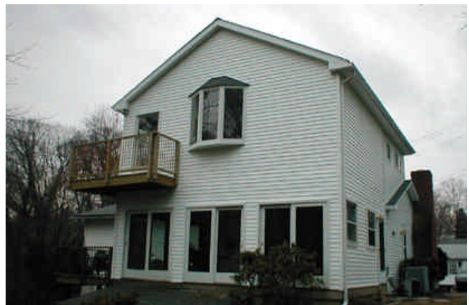
Rear yard elevation, after
