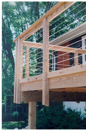
View of new deck railing
