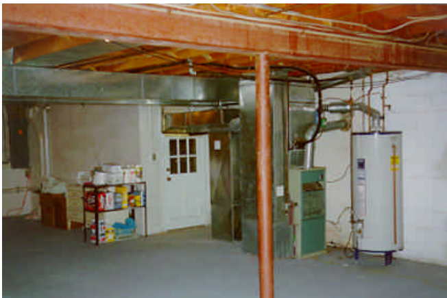
Unfinished basement, before
