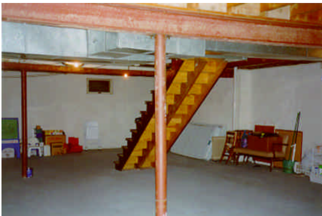
Unfinished basement, before
