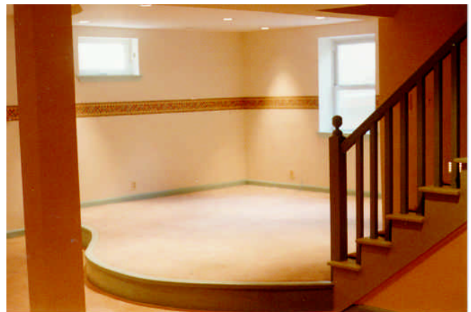
Refurbished stair with play stage and new windows
