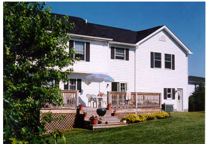
Addition seen beyond existing deck
