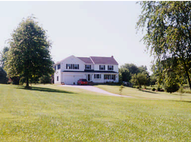
After addition with new access from front
